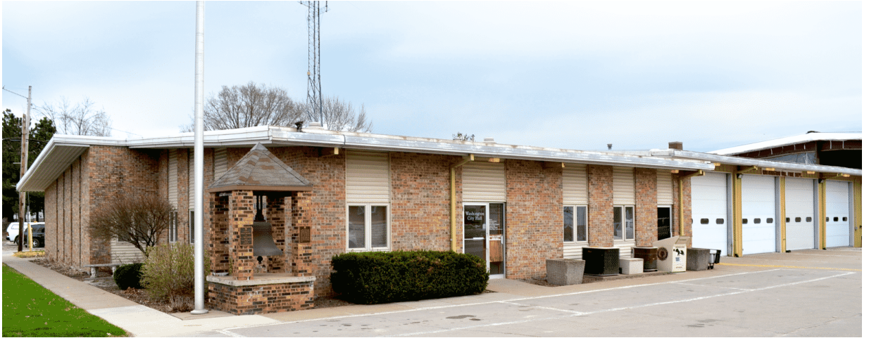
Before Renovation- City Hall, Police, Fire
