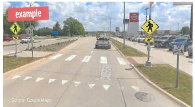
Example of an enhanced pedestrian crossing with RRFBs from Cedar Falls, Iowa.
