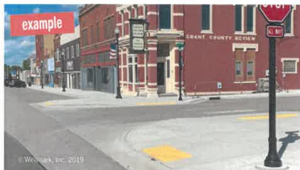
Example of a recently constructed bumpout in Milbank, South Dakota.
