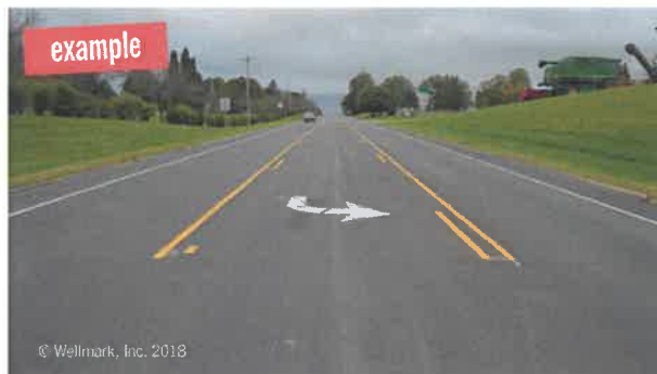
Example of a road diet with new three-lane striping completed as part of a resurfacing project on Iowa State Highway 9 in Waukon, Iowa.
