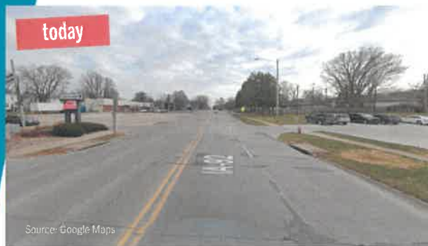
Highway 92 in Washington could benefit from a four-lane to three-lane conversion, also known as a road diet.
