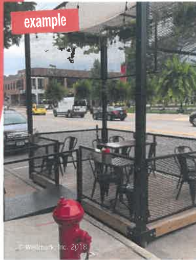
This parklet from Iowa City, Iowa was designed for easy removal during the winter months.
