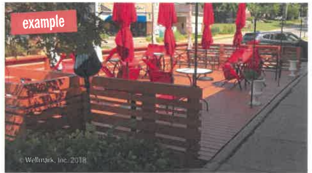
Example parklet constructed in front of a restaurant in Windsor Heights, Iowa.
