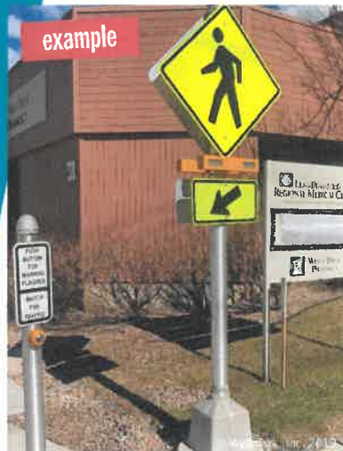
Enhanced pedestrian crossing with RRFBs like this example from Lead, South Dakota.
