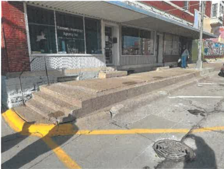
Figure 6. North of West Alley on South Iowa Avenue
