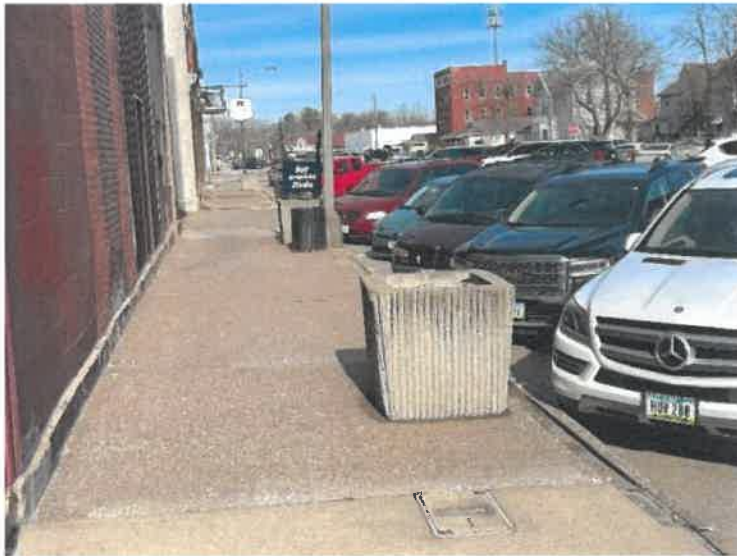
Figure 12. West Sidewalk of N. Iowa Avenue
