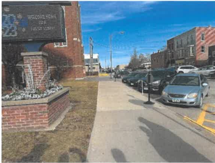
Figure 7. West Sidewalk on South Marion Avenue
