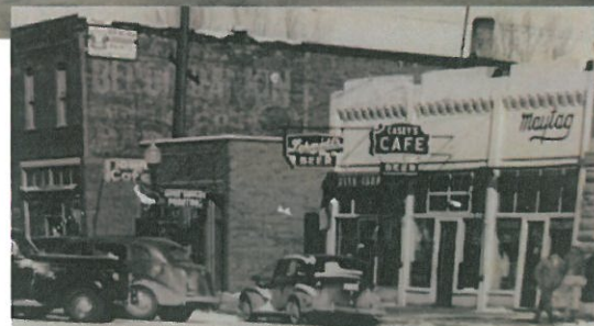
Historic image of the alley half of the building. (above) Sign is inspired by the "Casey's Café" historic sign.
