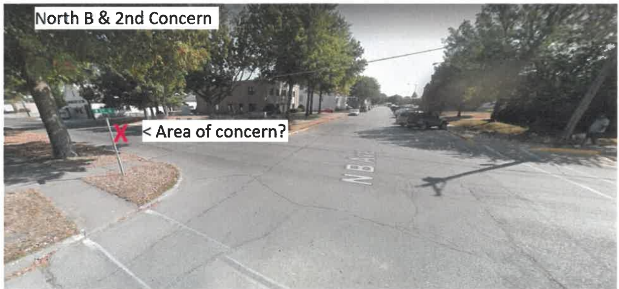
North B & 2 nd Street Concern (by County Communications Center)
