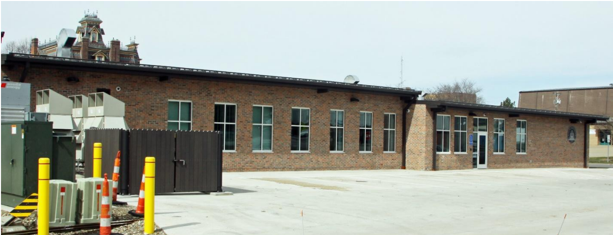
Rear of Building/ Staff Access
