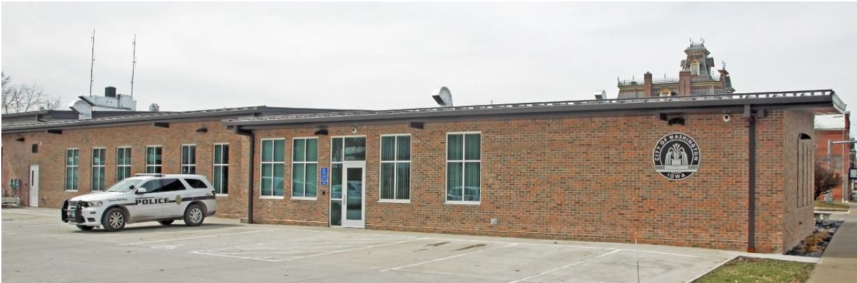
Rear of Building/Staff Access
