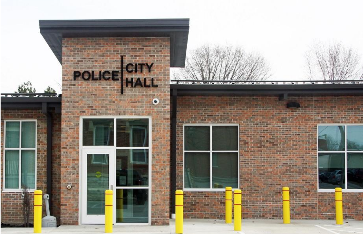
City Hall/Police Entry Vestibule
