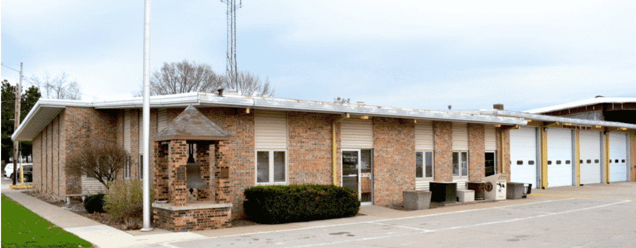
City Hall/Police/Fire- Before
