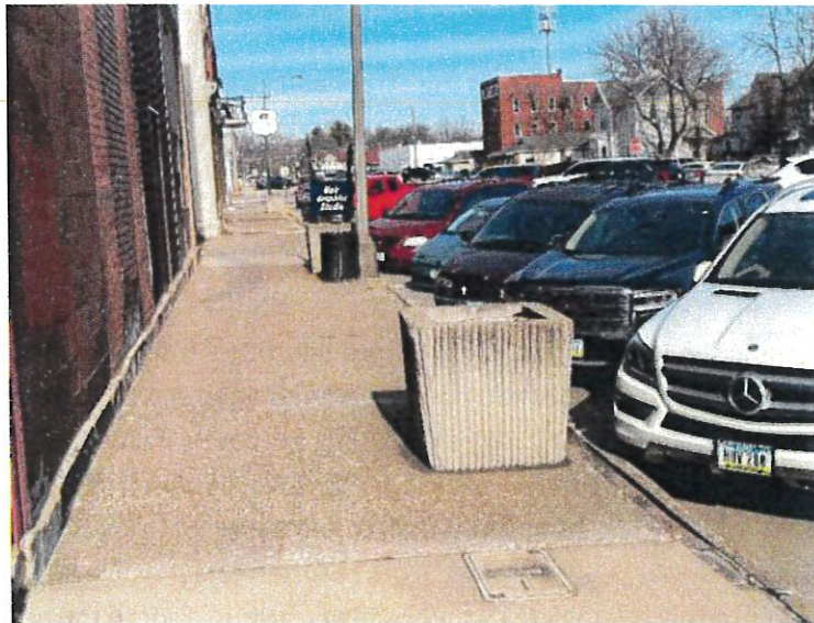
Figure 12. West Sidewalk of N. Iowa Avenue
