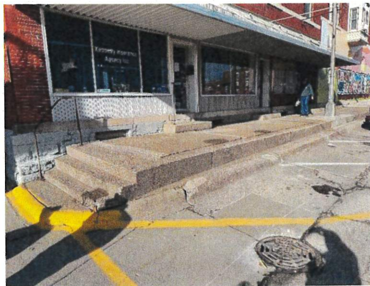
Figure 6. North of West Alley on South Iowa Avenue
