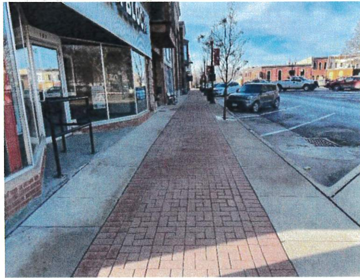
Figure 22. Typical Existing Downtown Sidewalk Paver Section
